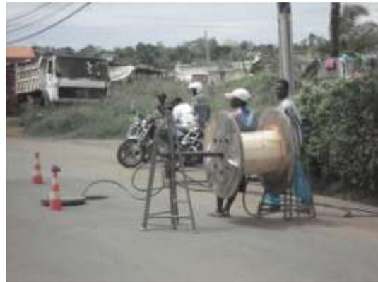
**Plate 10: Cable being placed under the road**
